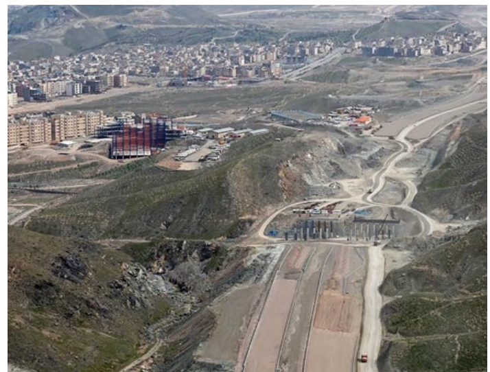
Fig. 5 A view of the studied project (south section)
