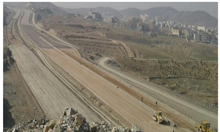
Fig. 4 A view of the studied project (north section)
